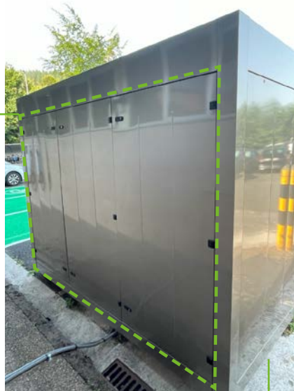
Dryer fume exhaust
